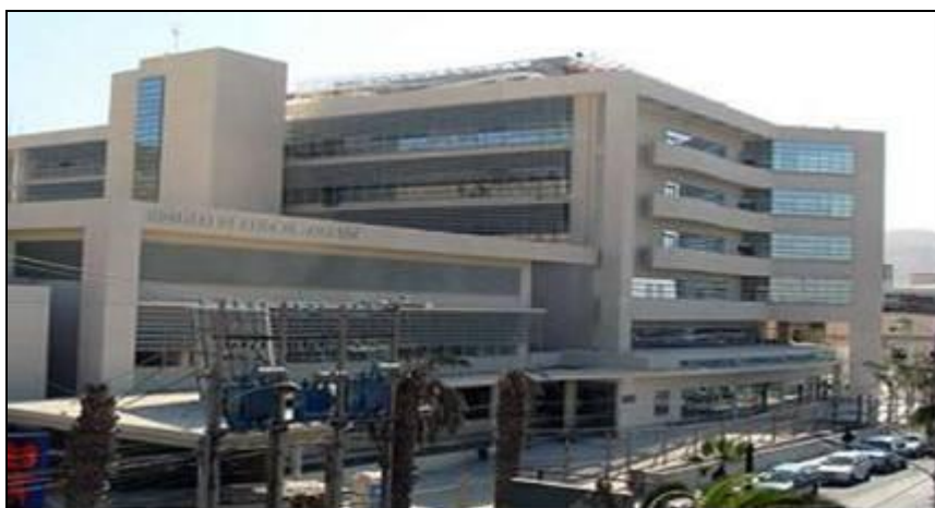
Fotografía 2-85. Hospital Regional de Arica, Dr. Juan Noe
